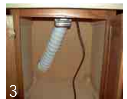
3 If the machine cannot be vented out the front of the cabinet. (See photo 1 and 2) Run the vent hose through side wall of the cabinet, keeping the length of the vent hose under 5' (1.52 meters) if at all possible. IMPORTANT: DO NOT vent the machine into a wall or closed space.
