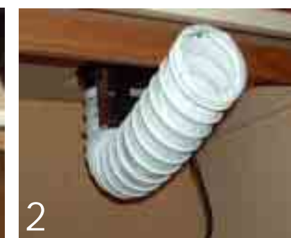
2 Make sure the vent hose is securely placed over the machines exhaust. Also make sure the vent hose is pulled taut and extends to the end of the cabinet. This will properly eject hot exhaust air and prevent recirculation.
